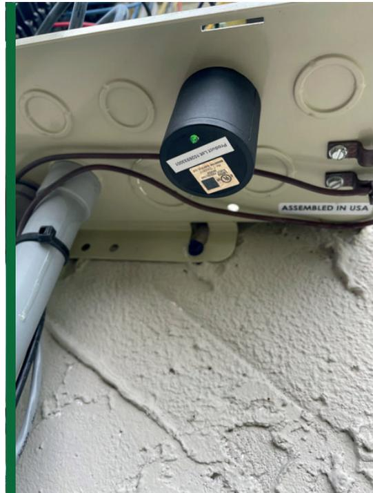
cannot put two wires into one breaker lug unless it was designed for that) you must remove the existing wire from the breaker then insert a small length of the same gauge wire. The existing wire and the TISPD lead can then be wire nudded to the small length of wire from the breaker. This is not shown below.
