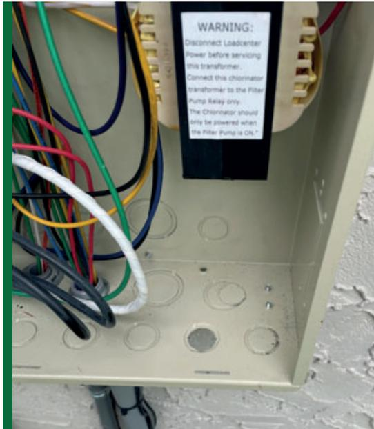
Insert the TISPD through the knockout hole and install the nut and washer, tighten hand tight. Do not overtighten and damage the plastic threads on the TISPD.
